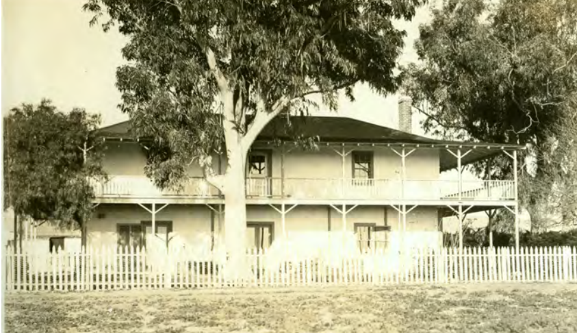
Figure 6: The south elevation of the Monterey block, ca. 1917. This was originally the primary façade of the house, and is the proposed location for the start of the interpretive trail.
