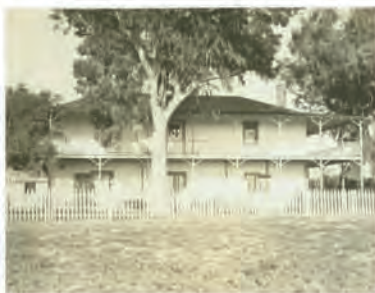
Above is an historic image of the two-story Monterey block porch, taken about 1920. Images like this one provided valuable information during the rehabilitation of the porch.
