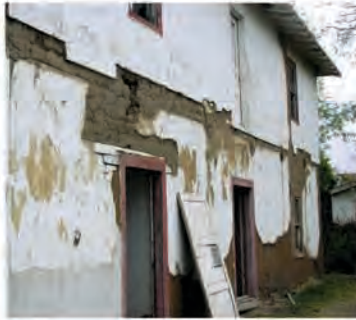
Two-story porches on the south, east, and west were lost in the 1980s, exposing perimeter walls to stucco loss and additional water damage.
