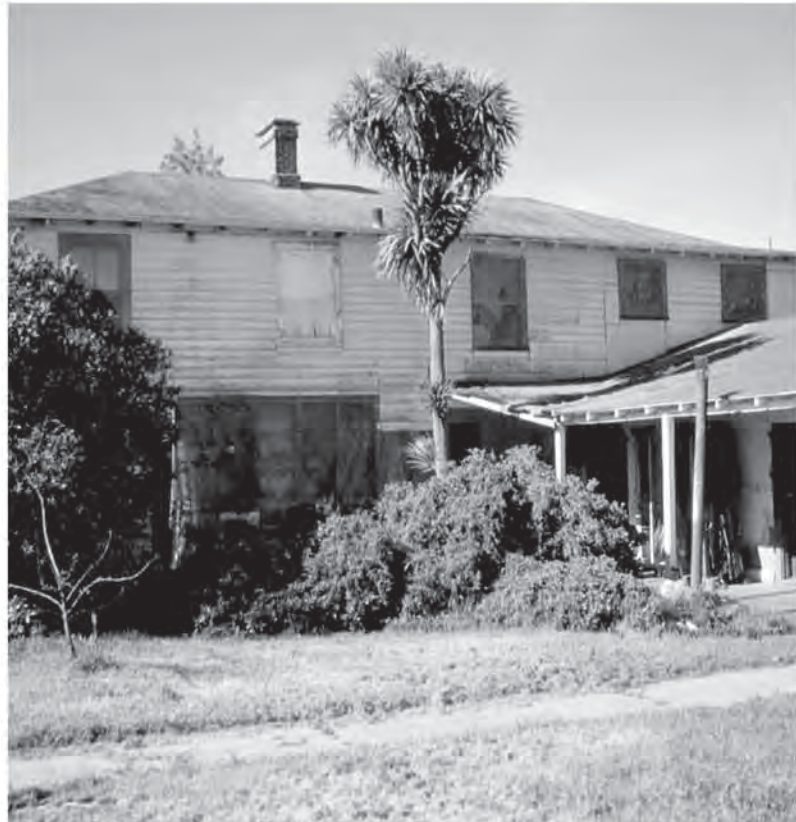
Two-story porches on the south, east, and west were lost in the 1980s, exposing perimeter walls to stucco loss and additional water damage.
